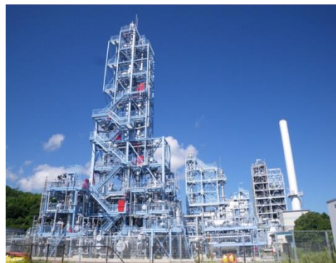
Physical absorption demonstration testing plant at the Wakamatsu Research Institute of Electric Power Development Co., Ltd. (J-POWER) (Source: Electric Power Development Co., Ltd. (J-POWER))
